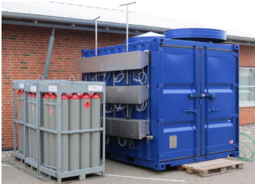
Figure 69. A 50 kW LT-PEMFC CHP hydrogen unit from Dantherm Power.
