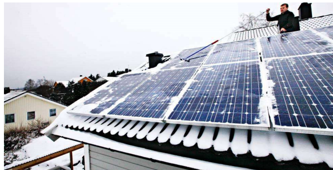
Figure 60. Snow being removed from solar panels mounted on a roof top in Norway.
