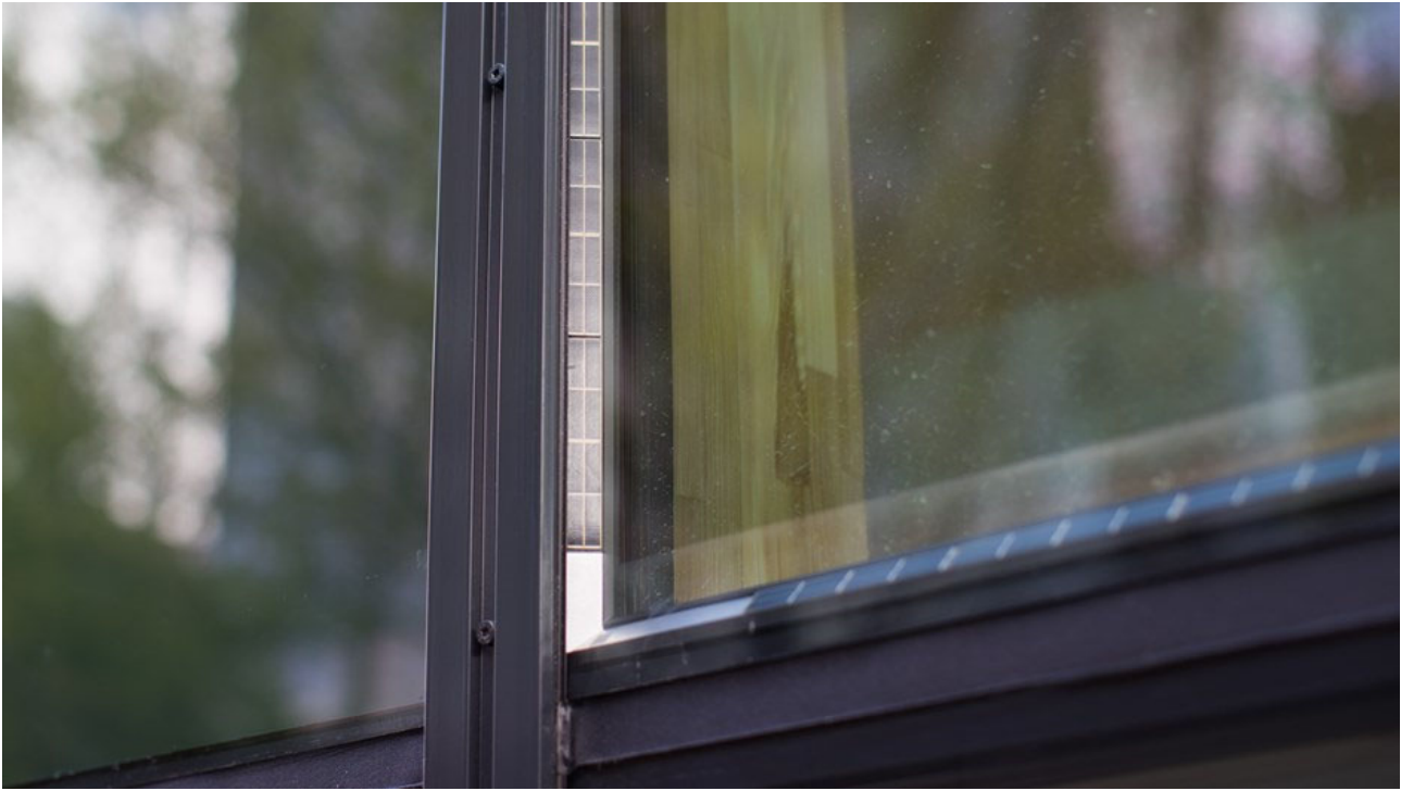
Figure 53. PowerWindow by Physee. Note the tilted PV at the spacer (photo: Jasper Juinen)
